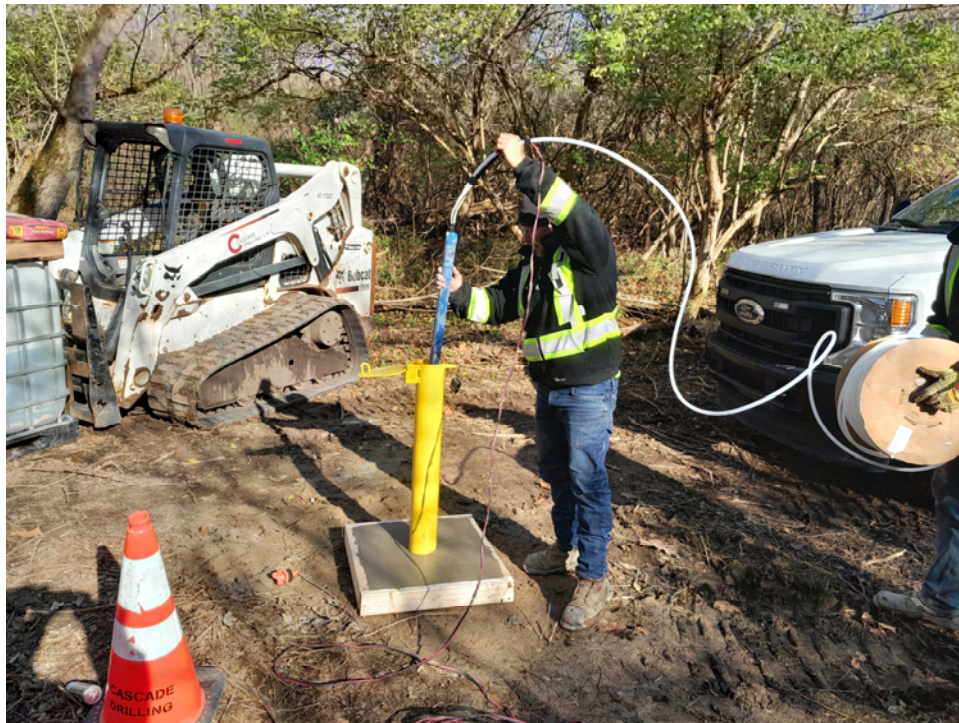
Figure 41. Monitoring well TRN-3 undergoing development via pump and surge method.
